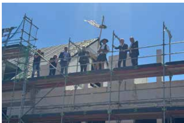
Bild: Airport Development A/S, Katrin Sobota
